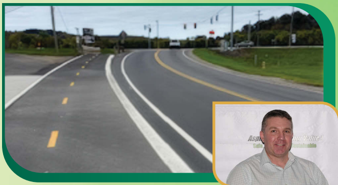
CONSTRUCTION OF SHARED-USE PATH ON C.R. 621 IN CANAL LEWISVILLE TO U.S. 36 IN COSHOCTON COUNTY ODOT District 5 THE SHELLEY CO.
