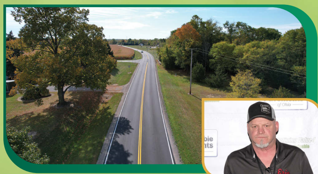
RESURFACING OF BERLIN ROAD FROM THE CITY OF HURON TO MASON ROAD IN ERIE COUNTY Erie County Engineer ERIE BLACKTOP INC.
