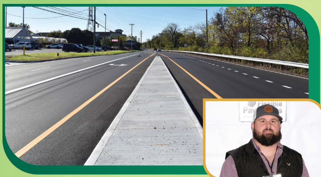
U.S. ROUTE 33 & HAYDEN RUN ROAD INTERSECTION IMPROVEMENT IN FRANKLIN COUNTY ODOT District 6 SHELLY & SANDS INC.
