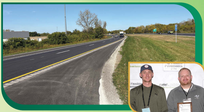
RESURFACING OF I-675 FROM CLARK COUNTY TO S.R. 235 IN GREENE COUNTY ODOT District 8 JOHN R. JURGENSEN CO.
