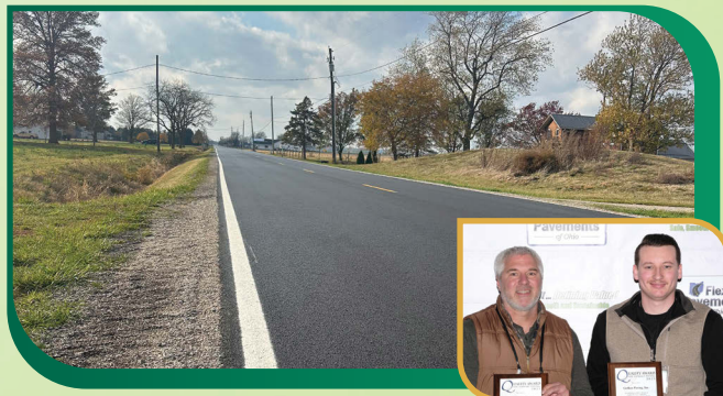
RESURFACING OF FIVE POINTS ROAD FROM S.R. 25 TO TRACY ROAD IN PERRYSBURG TOWNSHIP Perrysburg Township GERKEN PAVING INC.
