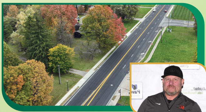
RESURFACING OF S.R. 422 FROM S.R. 616 TO THE COMMONWEALTH OF PENNSYLVANIA & S.R. 616 FROM NOTRE DAME DRIVE TO ROBINSON ROAD IN MAHONING COUNTY ODOT District 4 SHELLY & SANDS INC.
