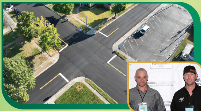
RESURFACING OF NORTH 3RD STREET, 4TH STREET, 5TH STREET & PARK AVENUE IN TIPP CITY City of Tipp City JOHN R. JURGENSEN CO.
