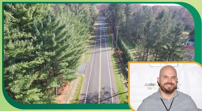
WIDENING & RESURFACING OF COREY ROAD FROM WHITEFORD ROAD TO MONROE STREET IN SYLVANIA TOWNSHIP Sylvania Township GERKEN PAVING INC.
