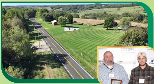
RESURFACING OF STATE ROUTE 95 FROM S.R. 60 TO SNOODY ROAD & S.R. 511 FROM S.R. 302 TO BASELINE ROAD IN ASHLAND COUNTY ODOT District 3 SHELLY & SANDS INC.
