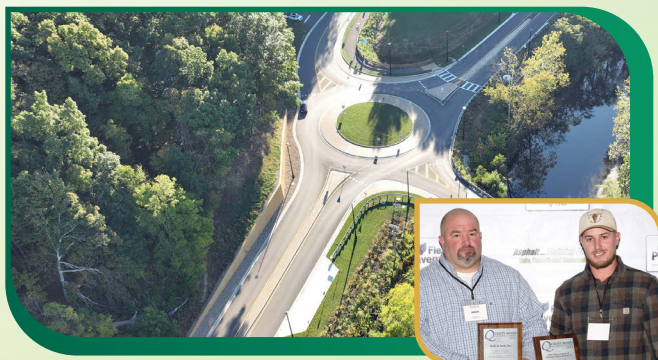
CONSTRUCTION OF A ROUNDABOUT AT S.R. 229, S.R. 308 & LAYMON ROAD IN KNOX COUNTY ODOT District 5 SHELLY & SANDS INC.
