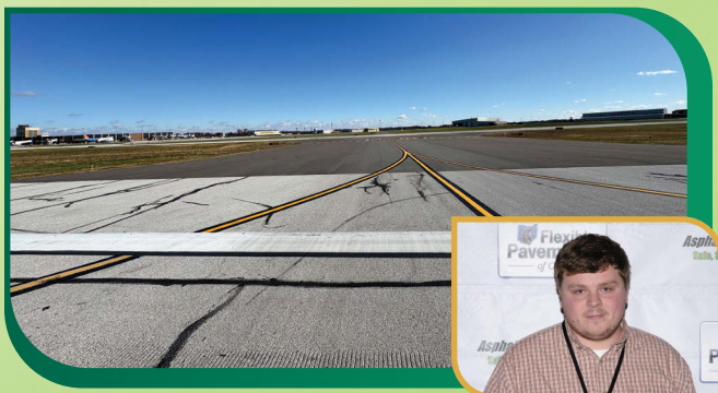
REHABILITATION OF TAXIWAY F AT THE AKRON-CANTON AIRPORT Akron-Canton Airport NORTHSTAR ASPHALT INC.
