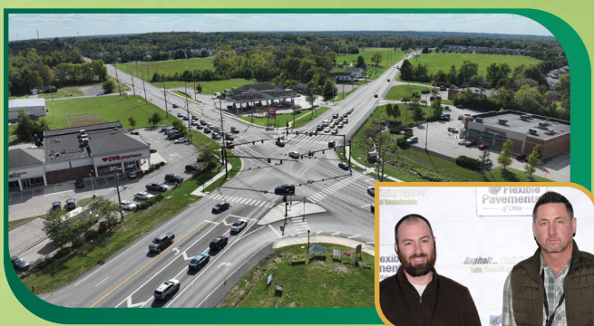
WIDENING & RESURFACING OF S.R. 48 IN WARREN COUNTY Warren County Transportation Improvement District & ODOT District 8 BARRETT PAVING MATERIALS INC.
