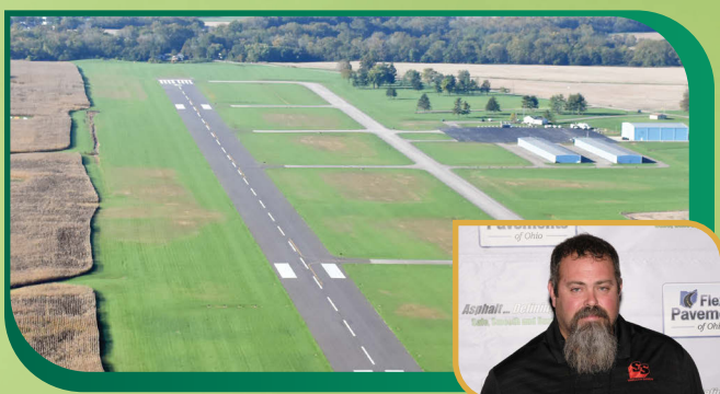
REHABILITATION OF RUNWAY AT THE MYRL SHOEMAKER ROSS COUNTY AIRPORT Ross County SHELLY & SANDS INC.
