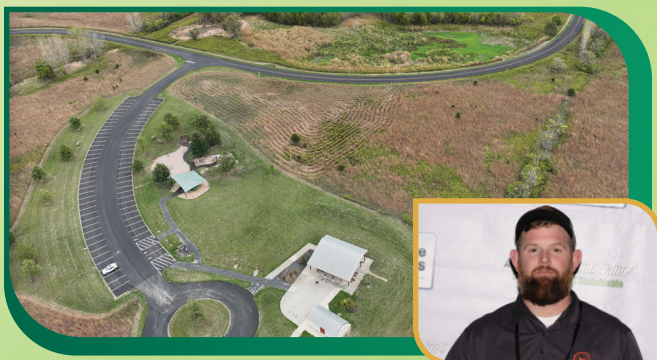
RESURFACING OF PARKING LOT AT PRAIRIE OAKS METRO PARK Columbus & Franklin County Metro Parks KOKOSING CONSTRUCTION CO. INC.
