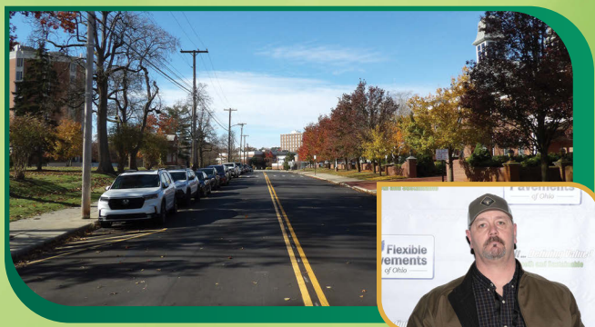
RESURFACING OF COLLEGE AVENUE FROM CENTER STREET TO CLAREMONT AVENUE IN THE CITY OF ASHLAND City of Ashland SARVER PAVING CO.
