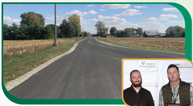
RESURFACING OF WELLS ROAD FROM EAST SHELBY ROAD TO S.R. 29 IN SHELBY COUNTY Shelby County Engineer BARRETT PAVING MATERIALS INC.
