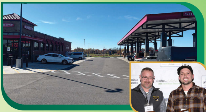
CONSTRUCTION OF PARKING LOT AT SHEETZ IN THE CITY OF FREMONT Sheetz Inc. EMPIRE PAVING LLC
