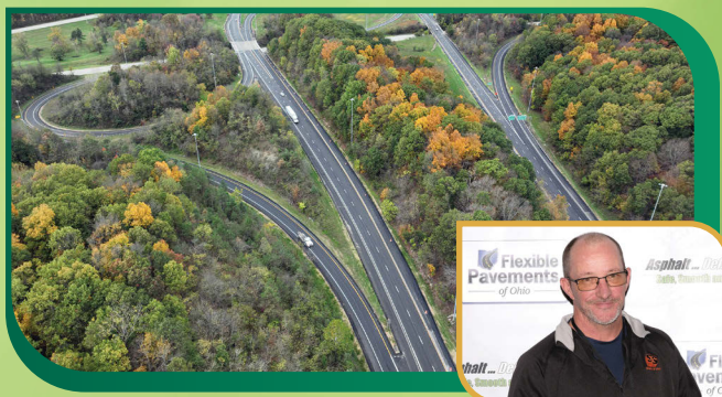
RESURFACING OF I-70 FROM I-77 TO S.R. 265 IN GUERNSEY COUNTY ODOT District 5 SHELLY & SANDS CO.
