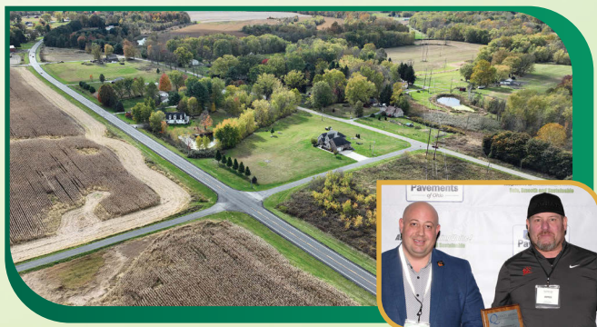
RESURFACING OF S.R. 534 FROM HALLOCK YOUNG ROAD TO MAPLE DRIVE IN TRUMBULL COUNTY ODOT District 4 SHELLY & SANDS INC.
