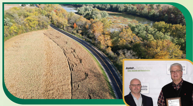
RESURFACING OF COUNTY ROAD 424 FROM HENRY COUNTY TO INDEPENDENCE ROAD IN DEFIANCE COUNTY Defiance County Engineer & ODOT District 1 GERKEN PAVING INC.
