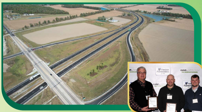
REHABILITATION OF U.S. ROUTE 24 FROM U.S. 127 IN PAULDING COUNTY TO BALTIMORE STREET IN THE CITY OF DEFIANCE ODOT District 1 GERKEN PAVING CO.
