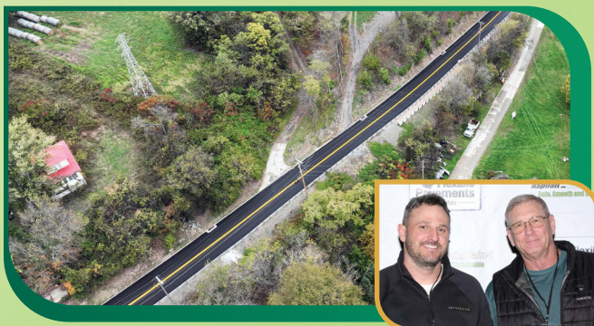
RESURFACING OF C.R. 26 FROM LINCOLN AVENUE TO C.R. 65 IN JEFFERSON COUNTY Jefferson County Engineer SHELLY & SANDS INC.
