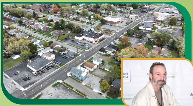
RESURFACING OF MAHONING AVENUE FROM MERIDIAN ROAD TO I-80 IN THE CITY OF YOUNGSTOWN City of Youngstown & ODOT District 4 SHELLY & SANDS INC.
