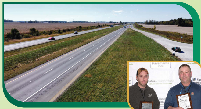
RESURFACING OF I-71 IN CLINTON AND GREENE COUNTIES ODOT District 8 JOHN R. JURGENSEN CO.
