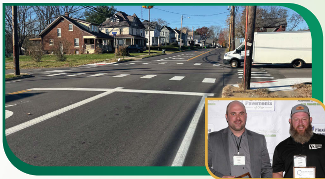
RESURFACING OF S.R. 172 FROM 32ND STREET TO S.R. 21 IN THE CITY OF MASSILLON ODOT District 4 NORTHSTAR ASPHALT INC.
