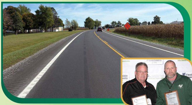
RESURFACING OF U.S. 68 FROM LOGAN COUNTY TO WASHINGTON AVENUE IN THE CITY OF URBANA ODOT District 7 JOHN R. JURGENSEN CO.
