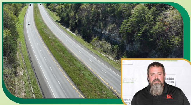
RESURFACING OF S.R. 35 FROM GALLIA COUNTY TO ORPHEUS ROAD IN JACKSON COUNTY ODOT District 9 SHELLY & SANDS INC.
