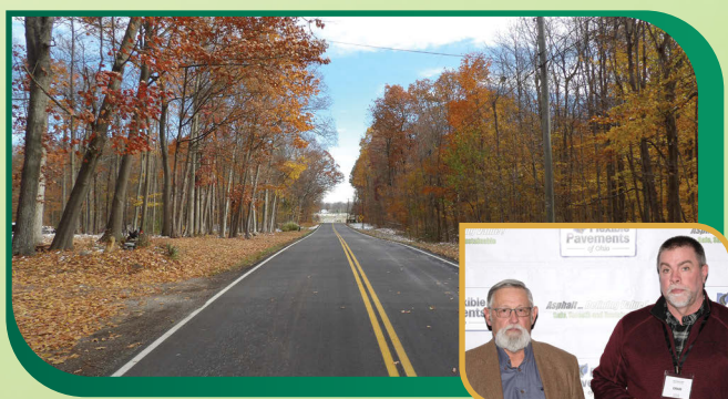
RESURFACING OF C.R. 620 FROM S.R. 511 TO S.R. 89 IN ASHLAND COUNTY Ashland County Engineer SARVER PAVING CO.
