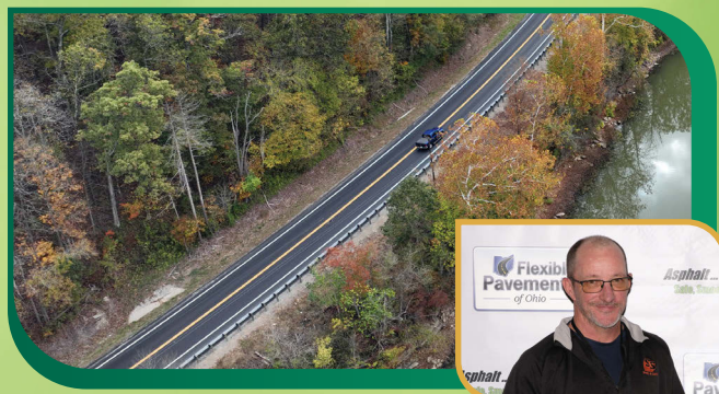
REHABILITATION OF S.R. 60 FROM MORGAN COUNTY TO DUNCAN FALLS IN MUSKINGUM COUNTY ODOT District 5 SHELLY & SANDS INC.
