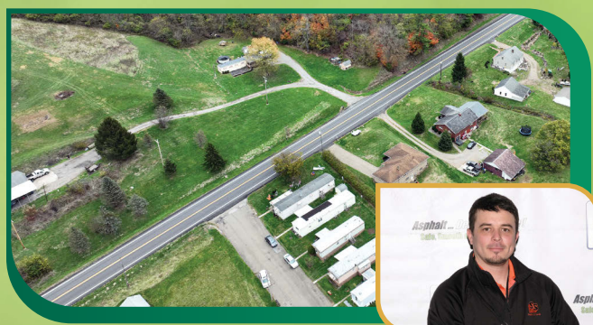
RESURFACING OF U.S. ROUTE 250 IN HARRISON COUNTY ODOT District 11 SHELLY & SANDS INC.
