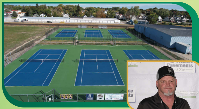
CONSTRUCTION OF TENNIS COURTS IN THE CITY OF SANDUSKY City of Sandusky ERIE BLACKTOP INC.
