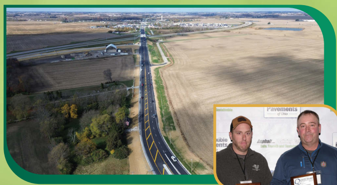
WIDENING OF S.R. 435 FROM U.S. 35 TO S.R. 729 & CONSTRUCTION OF A ROUNDABOUT AT S.R. 435 AND S.R. 729 IN FAYETTE COUNTY ODOT District 6 JOHN R. JURGENSEN CO.
