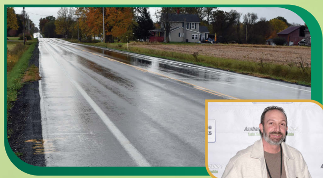
RESURFACING OF S.R. 45 FROM ASHTABULA COUNTY TO S.R. 87 IN TRUMBULL COUNTY ODOT District 4 SHELLY & SANDS INC.
