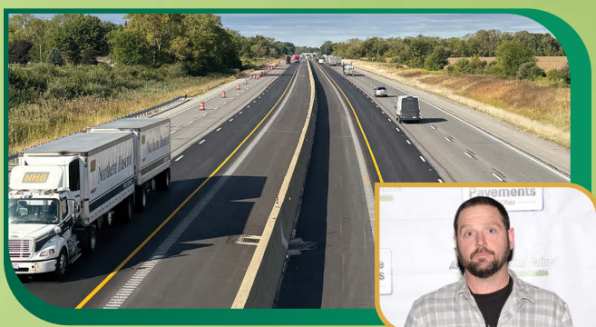
RESURFACING OF OHIO TURNPIKE FROM MP 118.8 TO MP 127.9 IN ERIE COUNTY Ohio Turnpike Infrastructure Commission KOKOSING CONSTRUCTION CO. INC.
