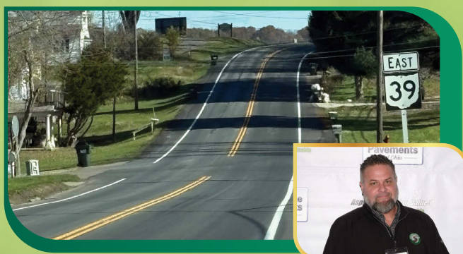
RESURFACING OF S.R. 39 FROM THE CITY OF NEW PHILADELPHIA TO THE VILLAGE OF ROSWELL IN TUSCARAWAS COUNTY ODOT District 11 SUPERIOR PAVING & MATERIALS INC.
