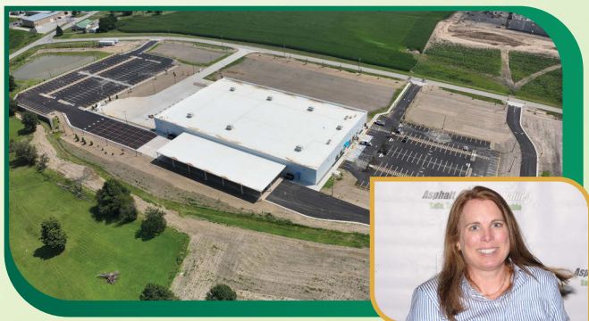
CONSTRUCTION OF PARKING LOTS & ROADWAYS AT AMAZON DISTRIBUTION CENTER IN THE CITY OF ASHLAND Walsh Construction Group LLC & Amazon KOKOSING CONSTRUCTION CO. INC.
