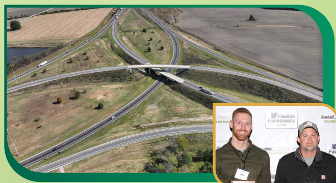
RESURFACING OF U.S. 23 & U.S. 30 IN WYANDOT COUNTY ODOT District 1 KOKOSING CONSTRUCTION CO. INC.
