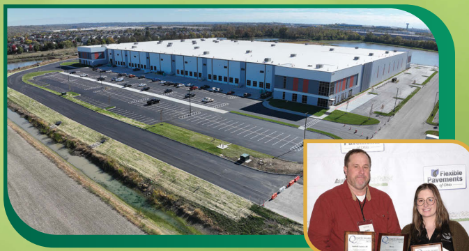
CONSTRUCTION OF PARKING LOT FOR FAIRFIELD LOGISTICS 1B IN THE CITY OF FAIRFIELD Fairfield Logistics 1B Merus SOUTHERN OHIO PAVING
