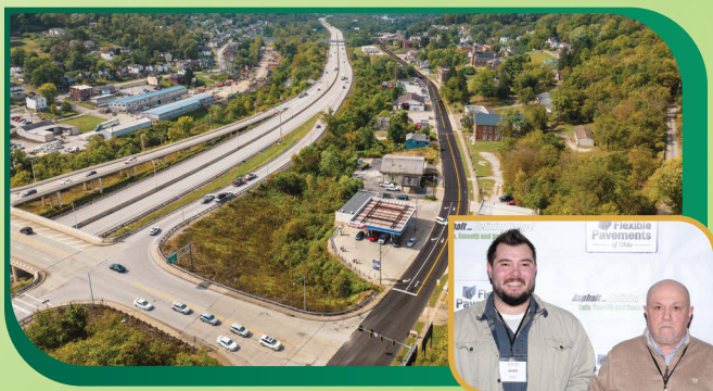
RESURFACING OF U.S. 250 & S.R. 767 IN BELMONT COUNTY ODOT District 11 NLS PAVING INC.
