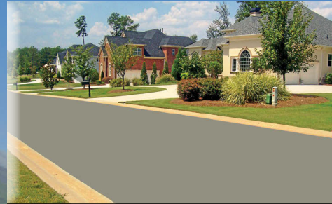
COOL PAVEMENT TECHNOLOGY
