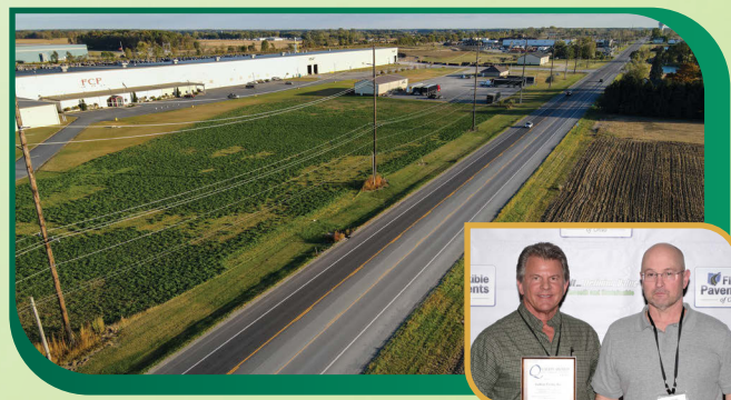
RESURFACING OF S.R. 109 FROM U.S. 20A TO U.S. 20 IN FULTON COUNTY ODOT District 2 GERKEN PAVING INC.
