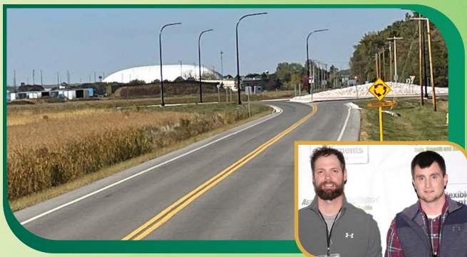
RESURFACING OF LIME CITY ROAD FROM U.S. 20 TO THE OHIO TURNPIKE & DEIMLING ROAD FROM CROSSROADS PARKWAY TO LIME CITY ROAD IN WOOD COUNTY Wood County Port Authority THE SHELLEY CO.
