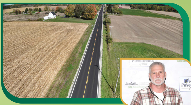
RESURFACING OF S.R. 423 FROM BARKS ROAD TO THE VILLAGE OF WALDO IN MARION COUNTY ODOT District 6 KOKOSING CONSTRUCTION CO. INC.
