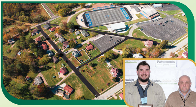
RESURFACING OF HOLMES AVENUE & MARTIN AVENUE IN THE VILLAGE OF CADIZ Village of Cadiz NLS PAVING INC.
