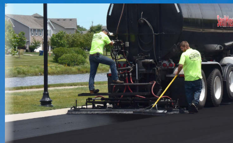
LIQUID ROAD SURFACE TREATMENT
