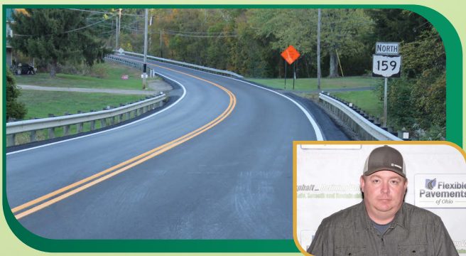
RESURFACING OF S.R. 159 FROM THE VILLAGE OF TARTLTON TO U.S. 22 IN FAIRFIELD COUNTY ODOT District 5 THE SHELLY CO.
