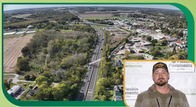
RESURFACING OF U.S. 30 IN WAYNE COUNTY ODOT District 3 KOKOSING CONSTRUCTION CO. INC.
