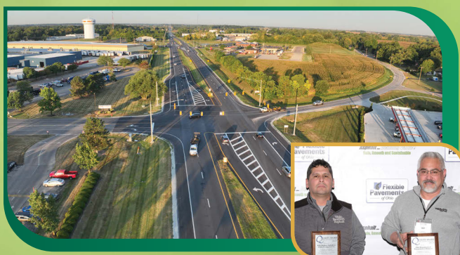
RESURFACING OF S.R. 55 FROM BARNHART ROAD TO GRANT STREET IN THE CITY OF TROY ODOT District 7 WALLS BROTHERS ASPHALT CO., A JOHN R. JURGENSEN CO.
