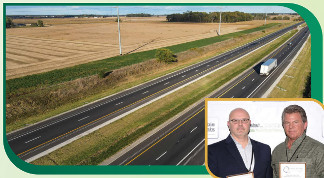
RESURFACING OF OHIO TURNPIKE FROM MP 43.0 TO MP 46.5 IN FULTON COUNTY Ohio Turnpike Infrastructure Commission GERKEN PAVING INC.
