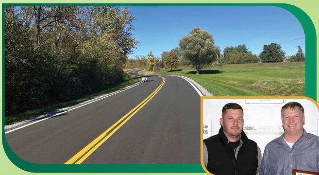
CONSTRUCTION OF ROUSH ROAD AT THE DODSON CREEK SOLAR IN HIGHLAND COUNTY Geronimo Power THE SHELLEY CO.
