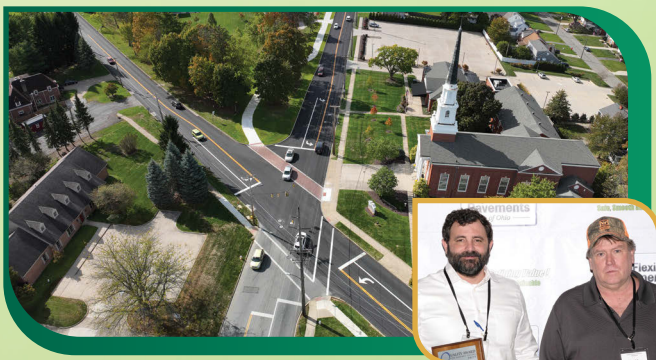
RESURFACING OF MILLSBORO ROAD & MARION AVENUE IN THE CITY OF MANSFIELD City of Mansfield KOKOSING CONSTRUCTION CO. INC.
