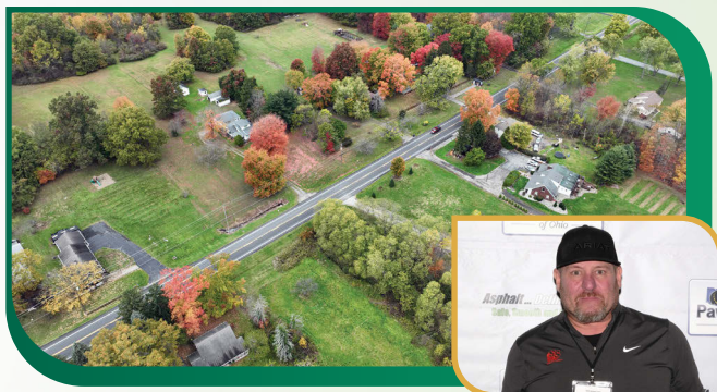
RESURFACING OF S.R. 7 FROM S.R. 82 TO DRAKE STATELINE ROAD IN TRUMBULL COUNTY ODOT District 4 SHELLY & SANDS INC.
