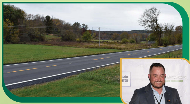
RESURFACING OF U.S. 22 FROM GUERNSEY COUNTY TO INDUSTRIAL PARK ROAD IN HARRISON COUNTY ODOT District 11 SHELLY & SANDS INC.
